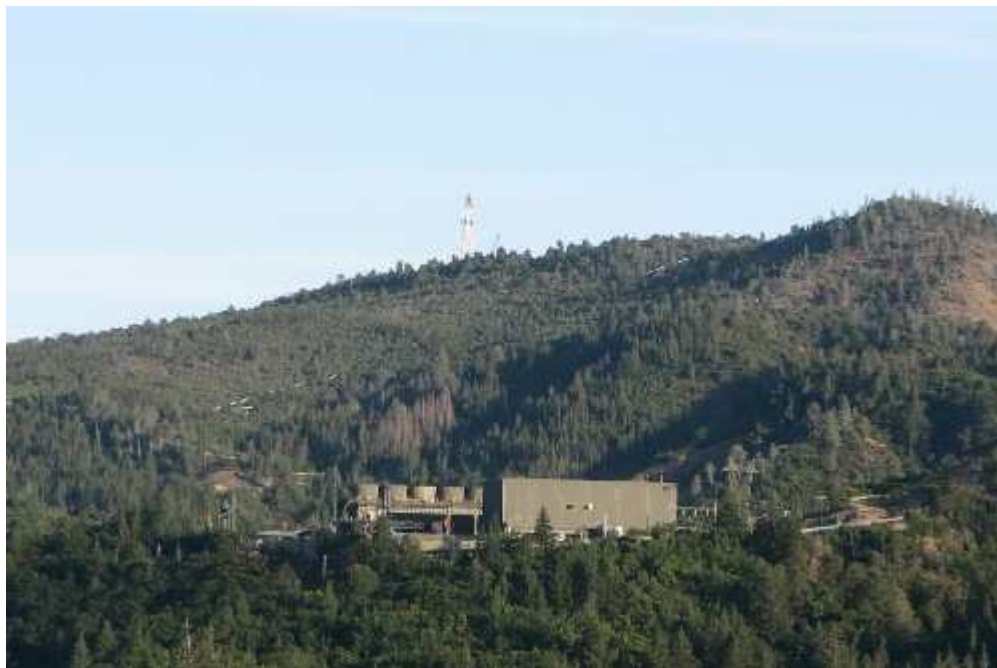
The AltaRock Energy derrick sits up high on a ridge at 3,150 feet. Photo courtesy of AltaRock.
